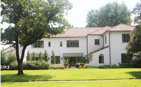
7218 Lakewood Blvd. Style: Mediterranean Revival
