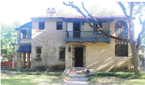
7226 Lakewood Blvd. Architect: Clifford D. Hutsell, 1932 Style: Monterey
