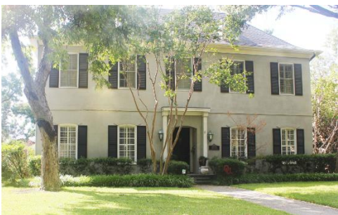
6936 Lakewood Blvd. Style: French Revival (Symmetrical)
